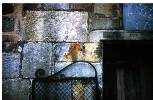
Fig. 1. Stone in situ externally at West Porch.
